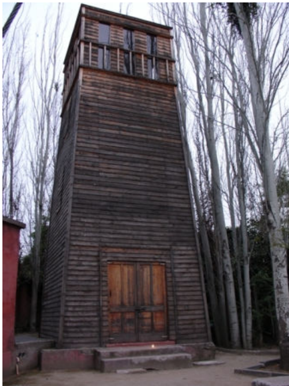
Photo 2, the reconstruction of the old water tower. Visitors can climb to the top floor, past the wooden isolation and torture cells.
